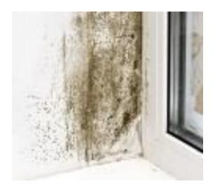
When applying another material atop concrete, there's an adhesive that goes in between. When the concrete is too moist, it can cause the adhesive to not work properly — making the top material loose and prone to shifting. As you already know, mold loves dampness and darkness. With a concrete structure that is too wet for completion, leaving it moist will allow the environment to generate mold. Furthermore, mold can continue to grow when it has a a fresh, wet underside of wood to keep it fed.
