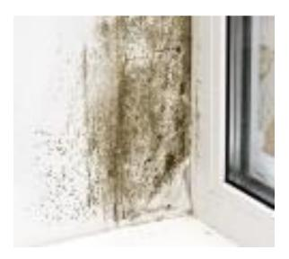
Using either pin-type meters or pin-less meters, detecting moisture under tile, wood floors and carpets is crucial to keeping the physical integrity of the location in solid, safe shape. Mold spores develop in wood starting at 20% moisture content, which is higher than drywall.
